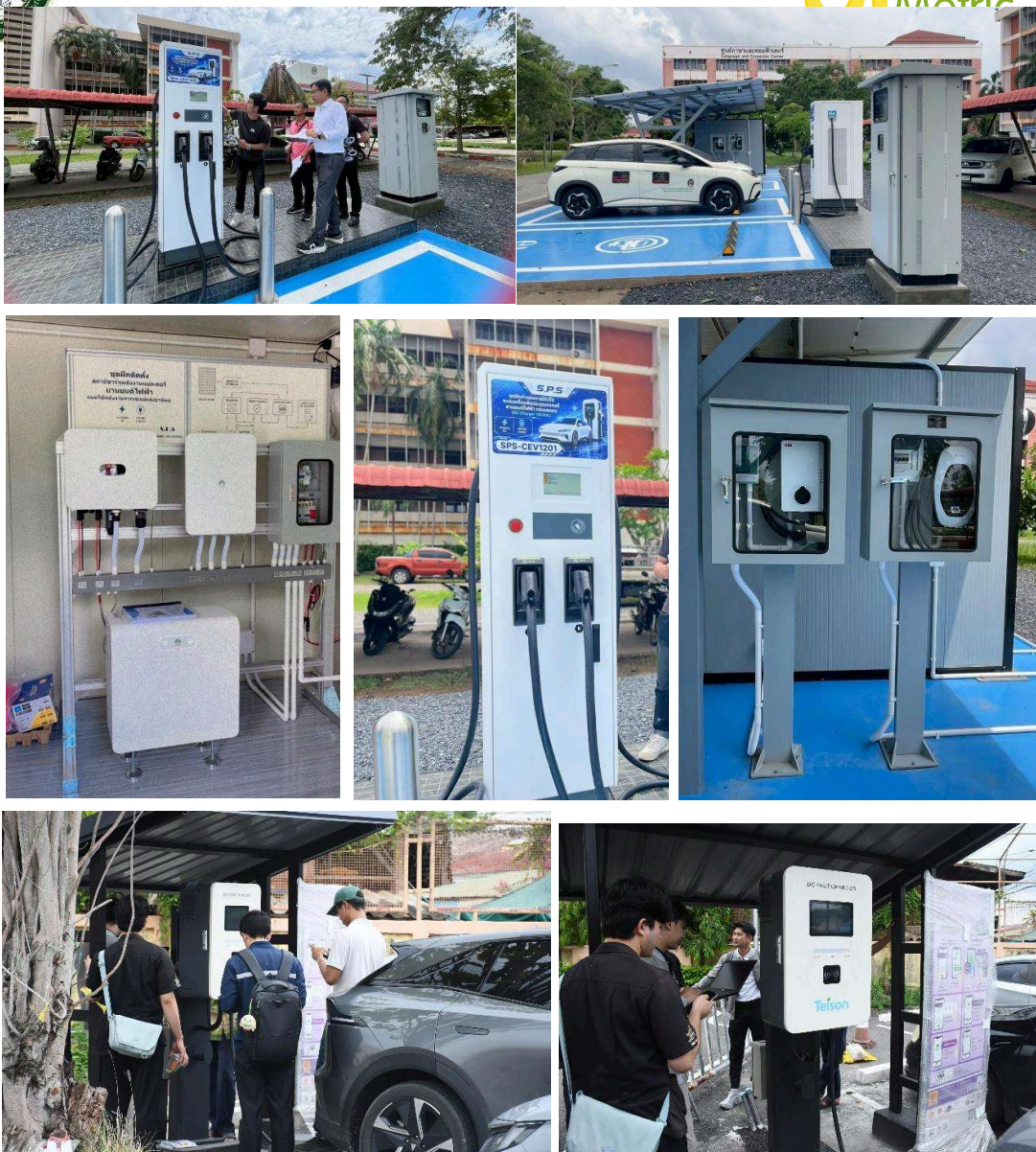
EV Charging Station Installation Project
